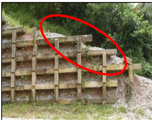
GAMBAR 15.11 Crib Wall Pecah
