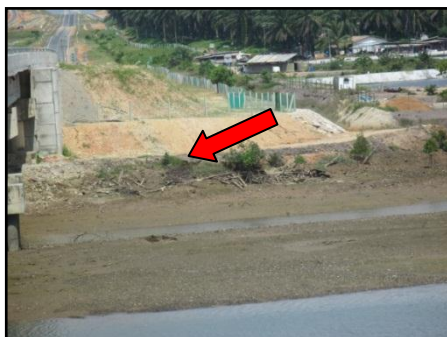
River Protection Belum Dibina Di Tebing Sungai Layau
