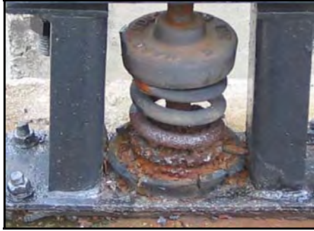
Spring Cooling Tower Stand Berkarat
