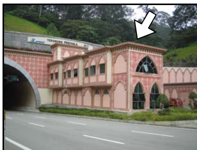
Control Room Penchala Link
