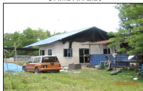
TKPM Serating, Marang - Bangunan Kekal Dibina di Lot 47 (05.09.2018)
