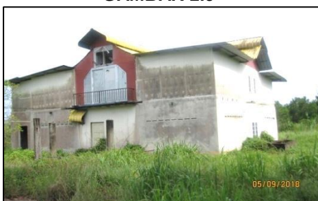
TKPM Serating, Marang - Bangunan Kekal Dibina di Lot 9 (05.09.2018)
