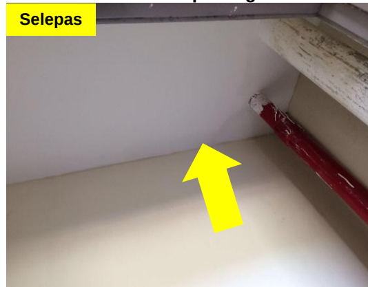
Gambar 1.28 Precast Lightweight Concrete Coping Telah Dipasang
