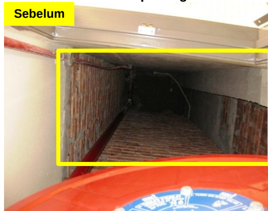
Gambar 1.27 Precast Lightweight Concrete Coping Tidak Dipasang
