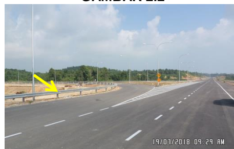
Phase 5 Stage 1 - Proposed Samalaju Boulevard Package 1 - Komponen Guardrail Siap Dibina (19.07.2018)
