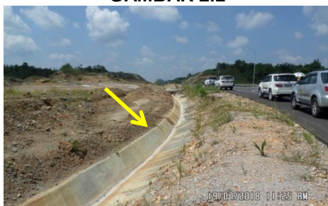
Phase 5 Stage 1 - Proposed Samalaju Boulevard Package 1 - Komponen Roadside Drain Siap Dibina (19.07.2018)
