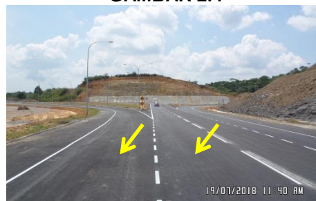
Phase 5 Stage 1 - Proposed Samalaju Boulevard Package 1 - Kerja Arrow Marking Belum Dilaksanakan (19.07.2018)
