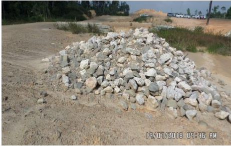
Phase 4 Stage 2 - Proposed Collector Road B2 - Block Stone yang Berada di Tapak Bina (19.07.2018)
