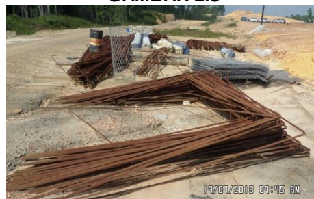
Phase 4 Stage 2 - Proposed Collector Road B2 - Cut & Bend Reinforcement yang Berada di Tapak Bina (19.07.2018)
