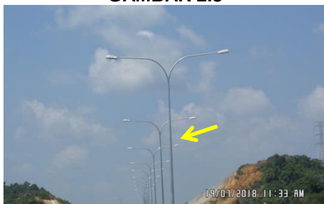
Phase 5 Stage 1 - Proposed Samalaju Boulevard Package 1 - Komponen Street Lighting Dalam Proses T&C (19.07.2018)
