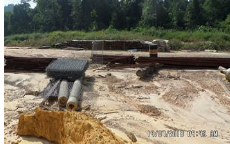
Phase 4 Stage 2 - Proposed Collector Road B2 - Gabion Mattress yang Berada di Tapak Bina (19.07.2018)
