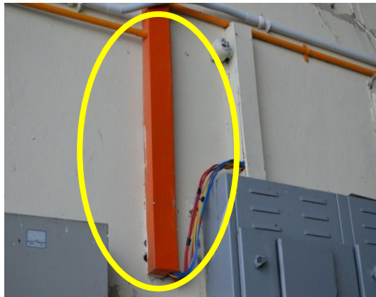
Gambar 3.3 Pemasangan Trunking Di Workshop
