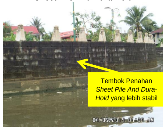
Gambar 1.7 Kualiti Estetik Tembok Penahan Sheet Pile And Dura-Hold
