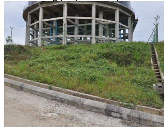
Gambar 3.23 Close Turfing (Slope Ground) Tidak Rata
