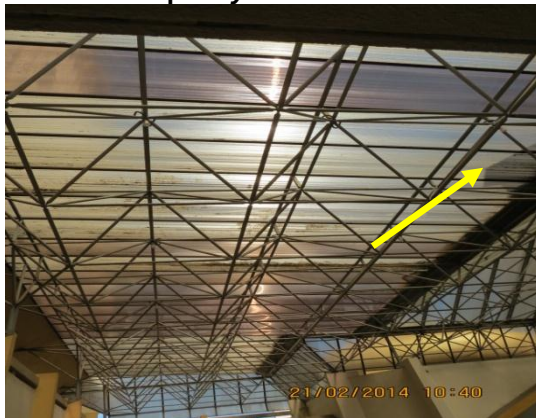
Gambar 6.5 Atap Polycarbon Bocor
