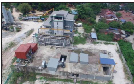
Loji Rawatan Kumbahan Serantau Batu - Main Process Plant Fasa 1 (Temporary Treatment Facilities/TTF) yang Beroperasi (Sumber: JPP)
