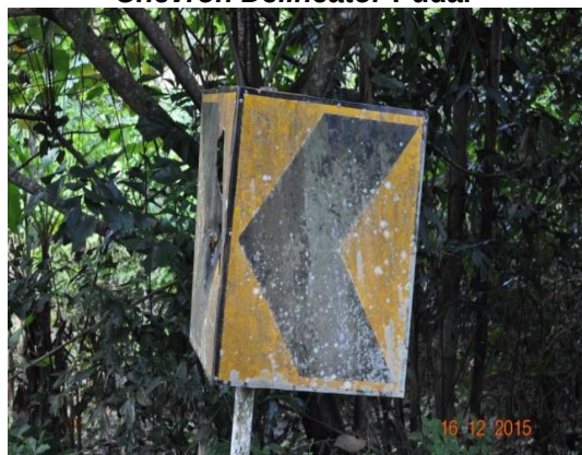
Gambar 1.8 Chevron Delineator Pudar
