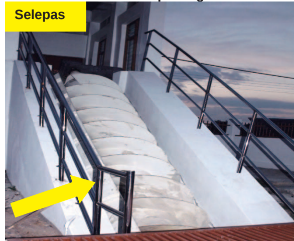
Gambar 4.15 Stainless Steel Handrailing Setelah Dipasang
