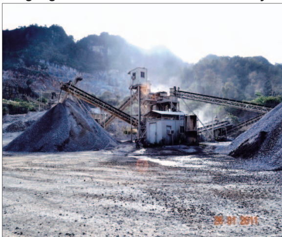
Gambar 8.1 Loji Crusher Pengangkutan Batu Melalui Sistem Conveyor
