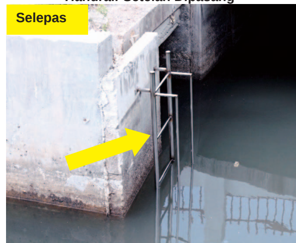
Gambar 4.13 Stainless Steel Cat Ladder With Handrail Setelah Dipasang
