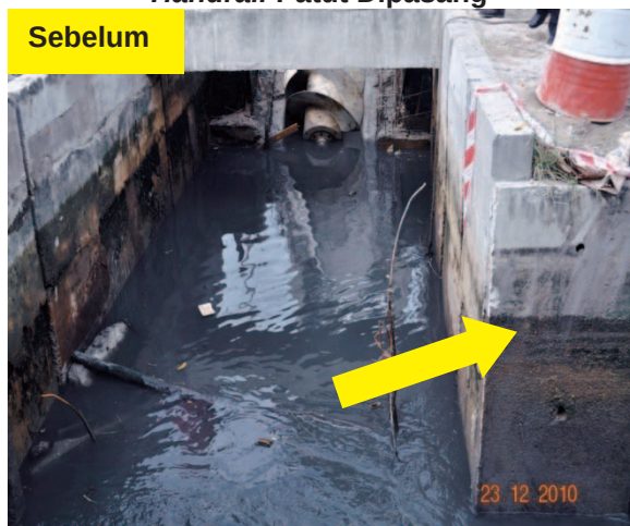
Gambar 4.12 Lokasi Stainless Steel Cat Ladder With Handrail Patut Dipasang
