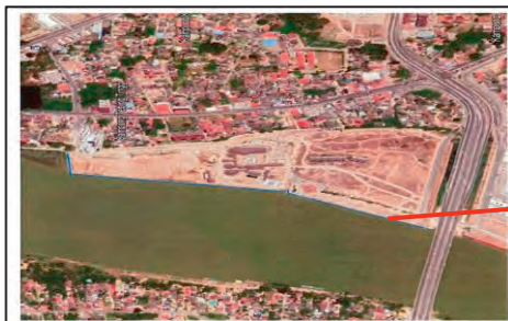
Gambaran Peta Retaining Wall di Zon B, - Pembinaan Retaining Wall (08.08.2019) (Sumber: UPEN)
